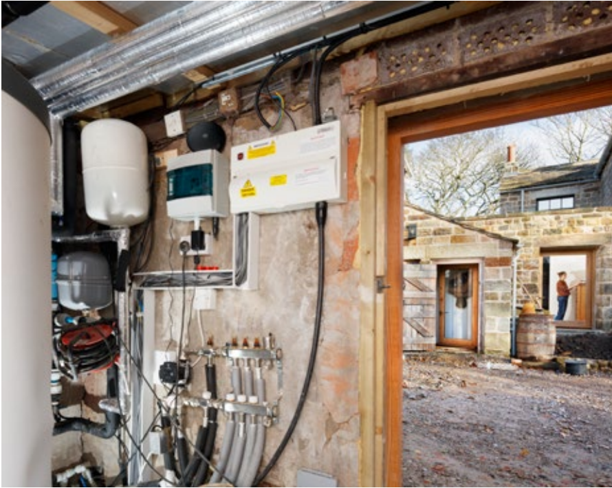
The mechanics of a ground source heat pump installed in a farm outhouse
