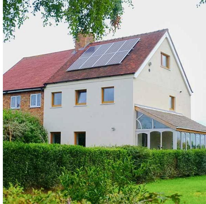
Retrofitting existing stock
