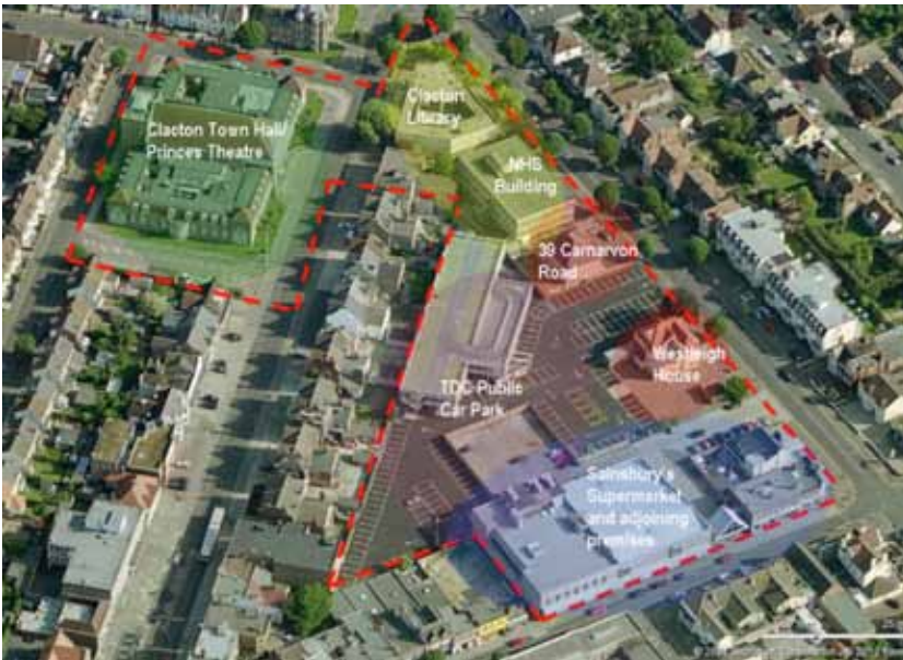
Existing building configuration on proposed campus site in Clacton, Tendring District, Essex. (Source Tendring DC)
