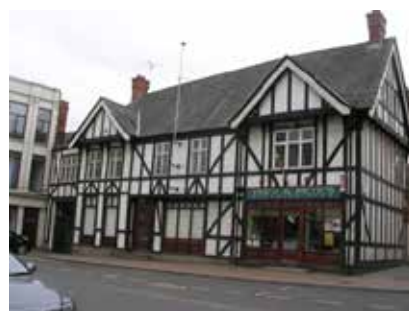
Part of 18 Bridge Street Banbury
