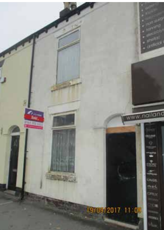
343 Chorley Road - a long term empty property compulsorily purchased
